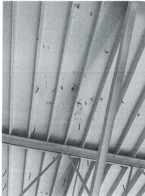
Photo Description: SW Corner, Underside: Metal corrosion due to roof leak
