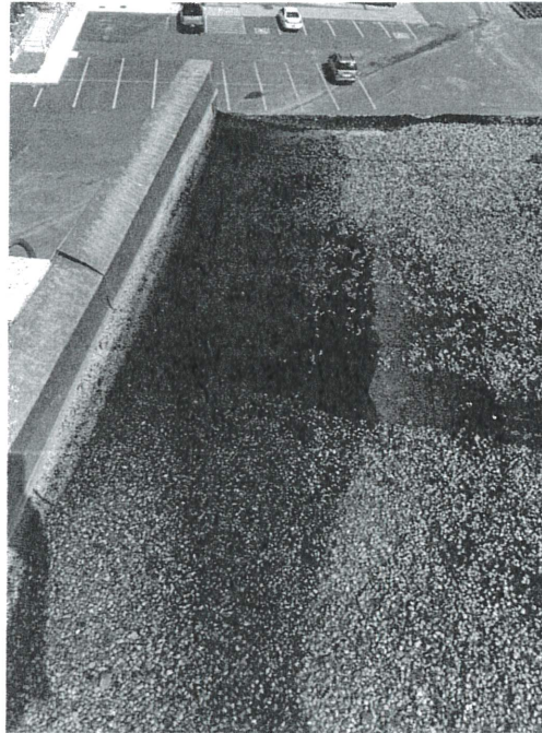
Photo Description: NW Corner of Roof: Damaged flashing and ponding water
